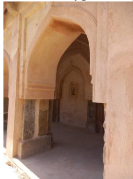
Fig.45 – Octagonal Stone Pillars are used. Source-Author
