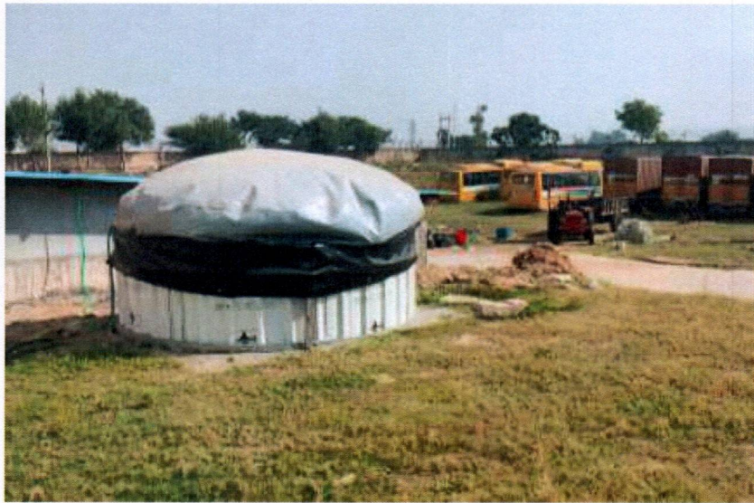
Figure 16 Bio Gas Plant
