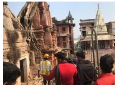
Fig. 4. Students at the transformational project of Kashi Vishwanath Temple at Varanasi (Source: Author).
